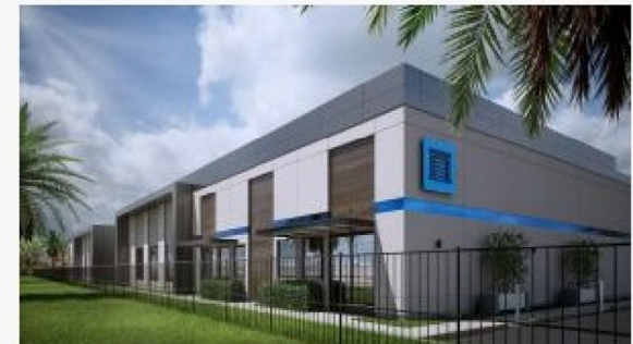
Luxury Warehouse Development Lakeland FL
